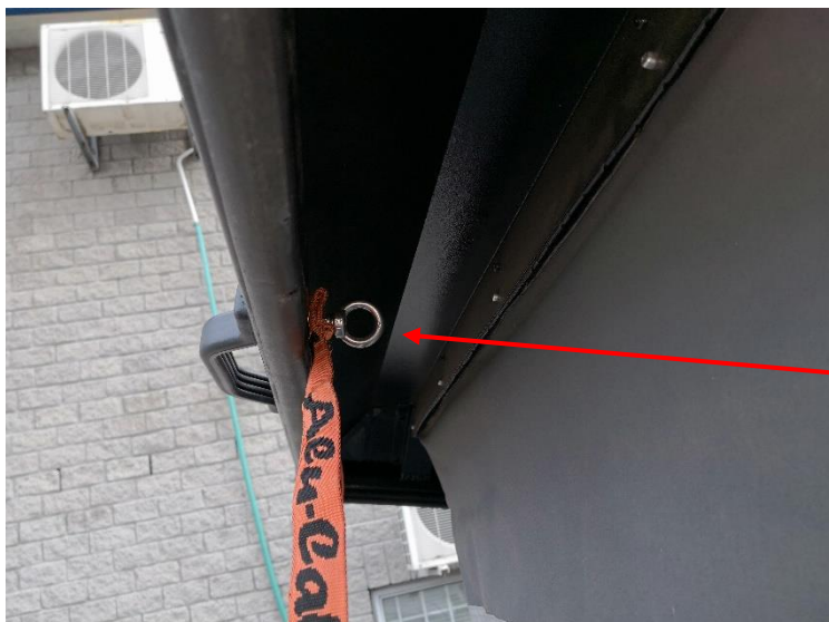
M6 Eye nut & Cam buckle strap with M6 eye nut fastened in the middle.
