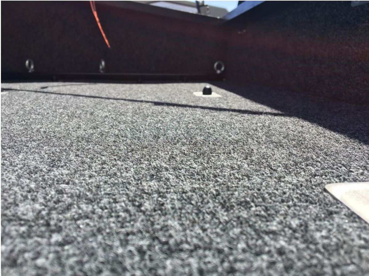
Figure 14: Completed Roof Box Securely Fastened
