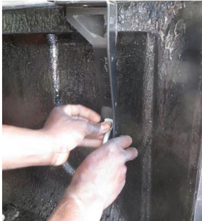
Figure 8: Aligning the Rear Support Bracket
