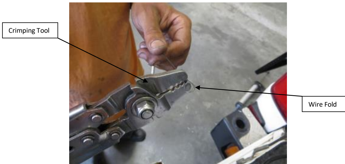
Figure 13: Crimping wires together
