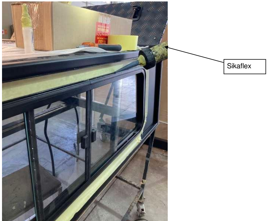
Figure 13: Add Sikaflex/Sealant.
