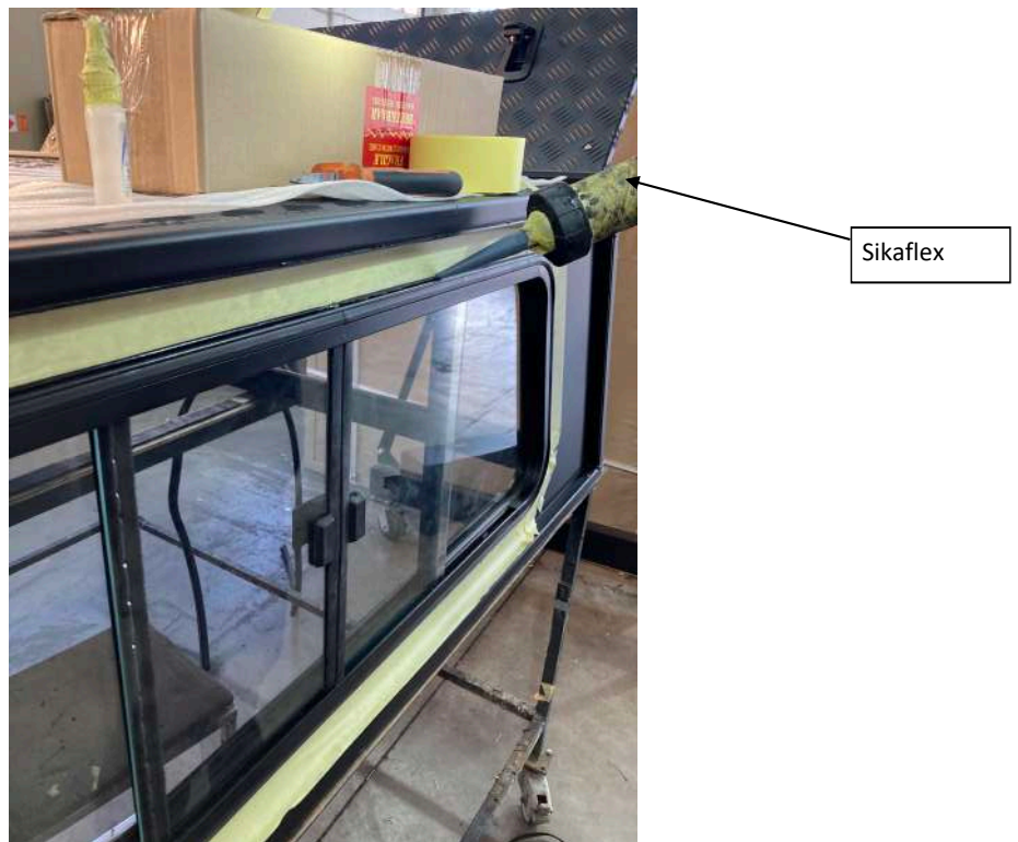
Figure 17: Add Sikaflex/Sealant.
