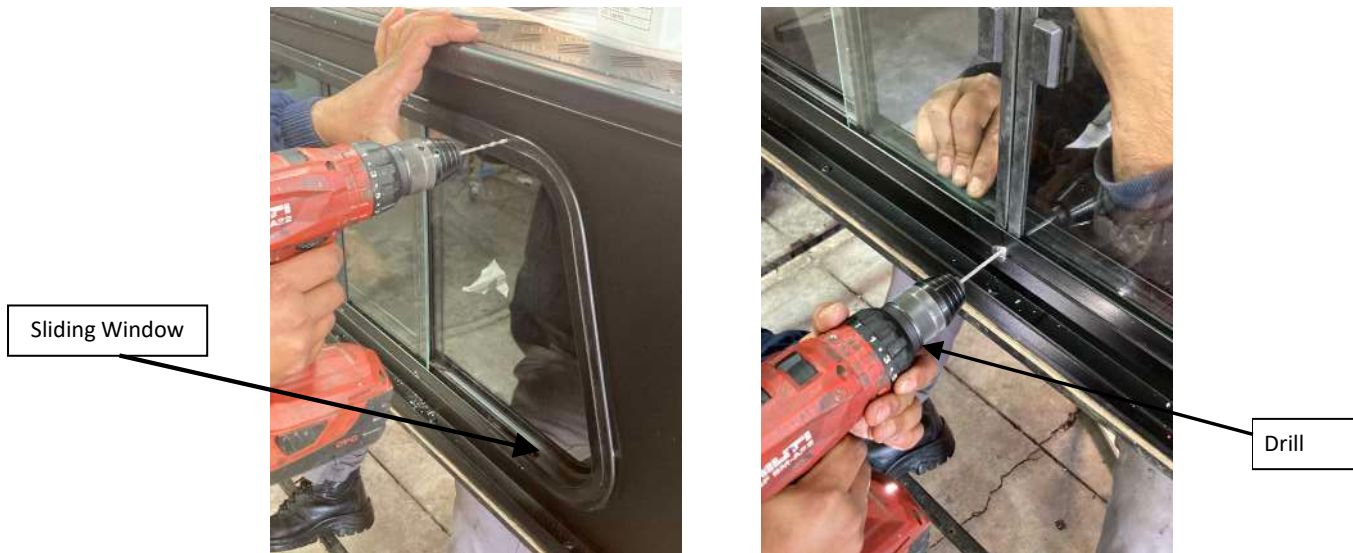
Figure 7: Drilling the holes to place rivets
