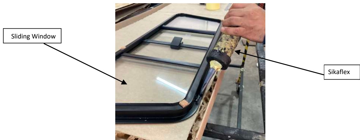
Figure 9: Add Sikaflex/Sealant to inside of window.
